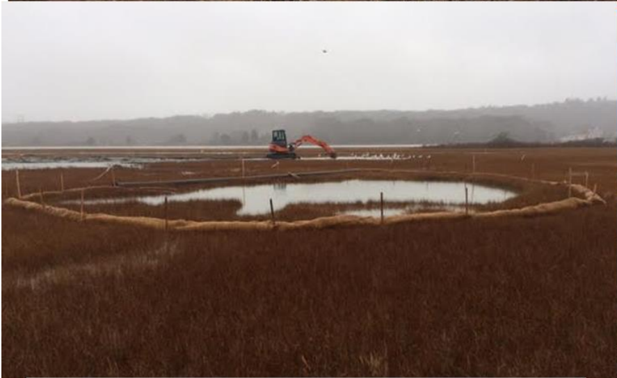
Before dredge, South Middlebridge.
