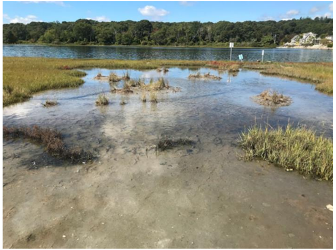
Drainage and microtopography installed
